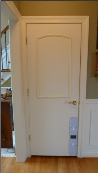
Step 6 – Align installation template bottom of door
