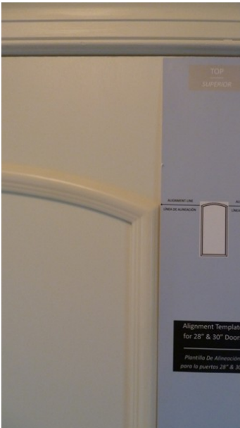
Step 5 – Align and place upper frame on door
