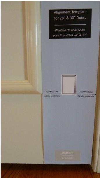
Step 7 – Align and place lower frame on door
