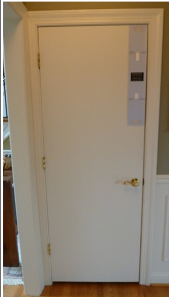
Step 4 – Align installation template on top of door
