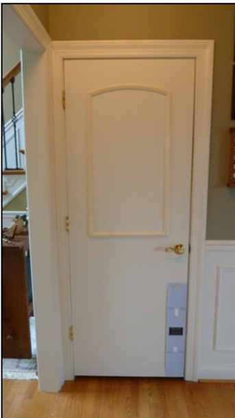
Step 6 – Align installation template bottom of door
