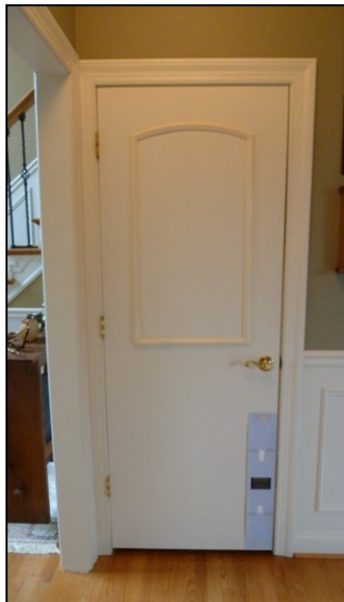
Step 6 – Align installation template bottom of door
