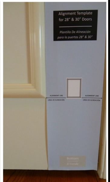
Step 7 – Align and place lower frame on door
