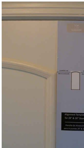
Step 5 – Align and place upper frame on door
